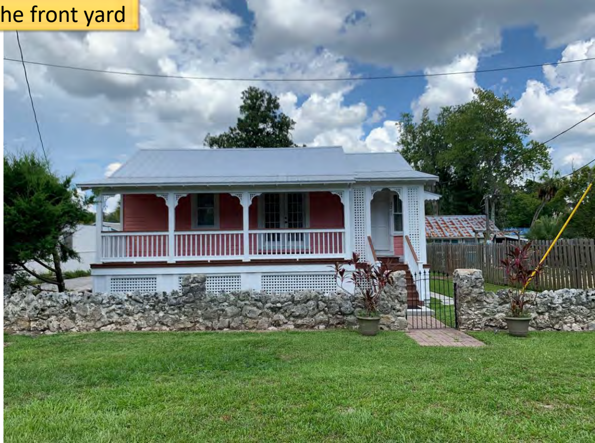
Nearby house with 40" wall lining street in front yard
