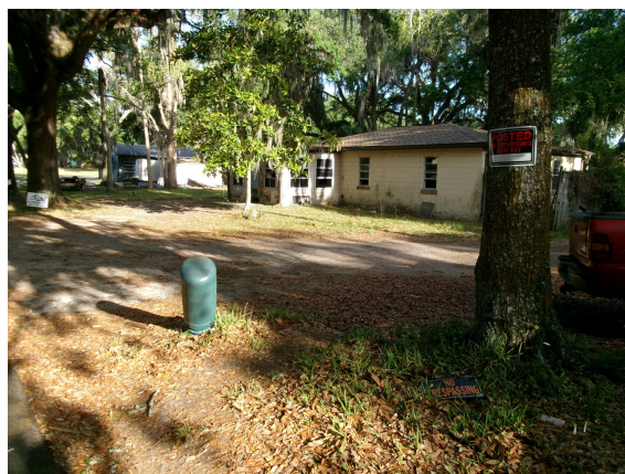
Existing SFR on NE 5 th Terr (west of site)
