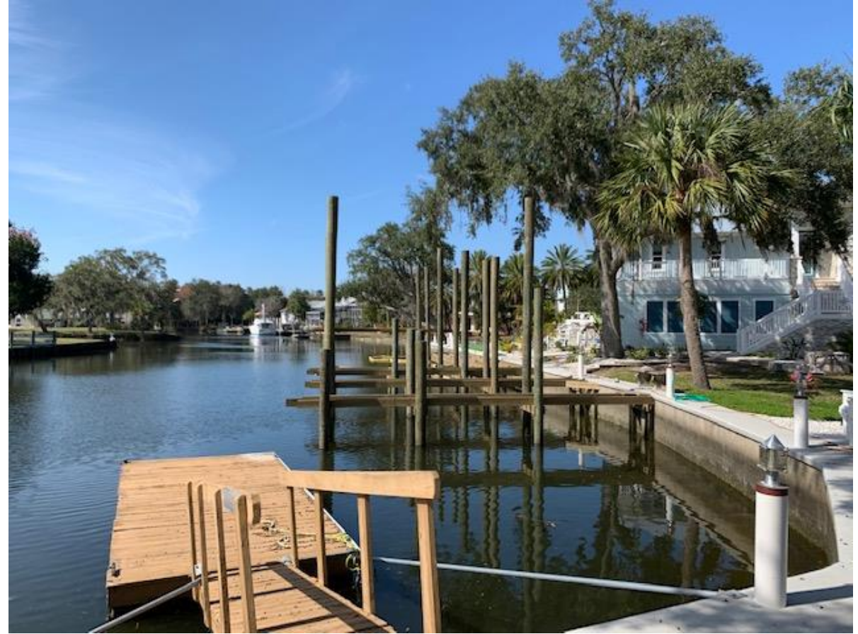
Proposed dock and boathouse – part of the requested variance – viewed from the east – southern property line
