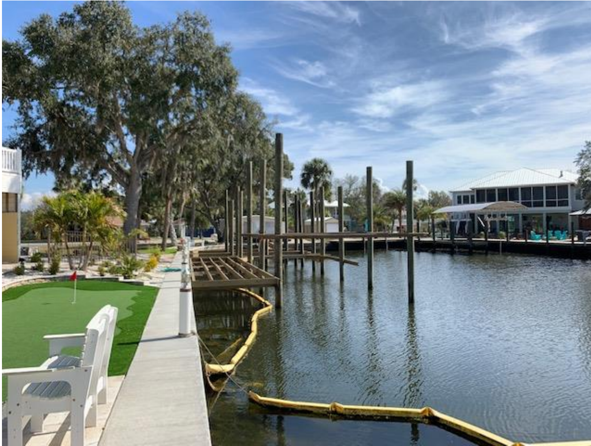
Proposed dock and boathouse – part of the requested variance – view from the west
