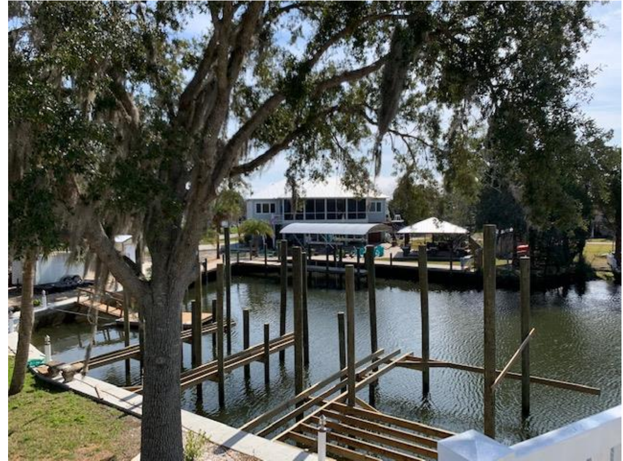
Proposed dock and boathouse – part of the requested variance – view from the house's balcony (north side)
