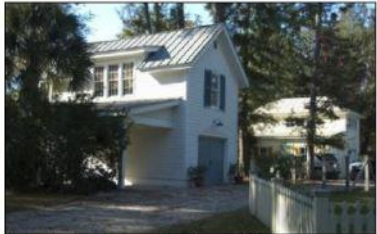
One-and-a-half-story carriage house with living area over the garage and an adjacent carport.
