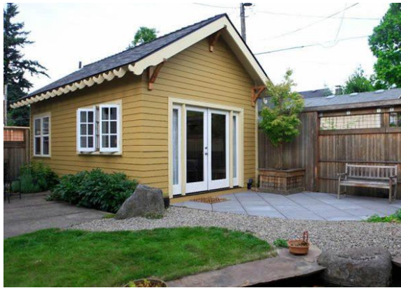
One-story carriage house – no garage.
