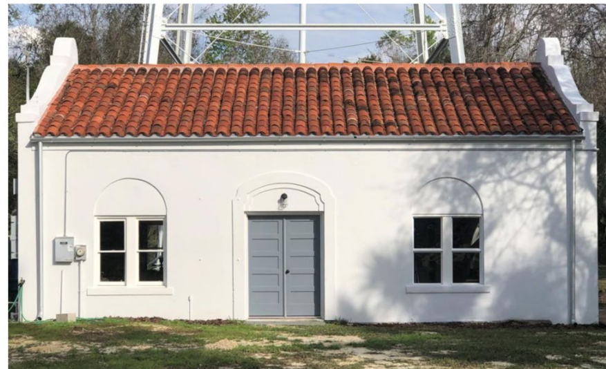
Front of Pumphouse After Refurbishment
