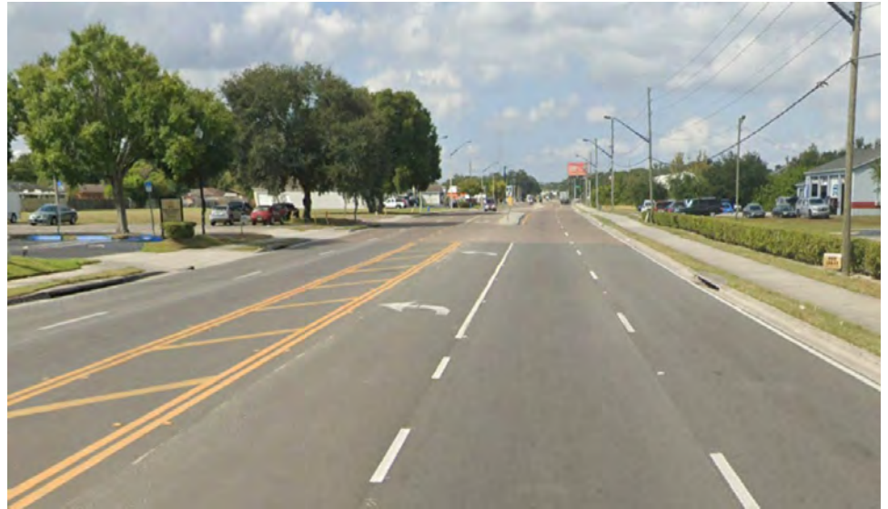
Above: SR-438 approaching Winter Garden. Below: Plant Street in Winter Garden
