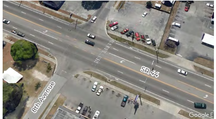
Existing conditions at the intersection of SR 44 with 8th Avenue
