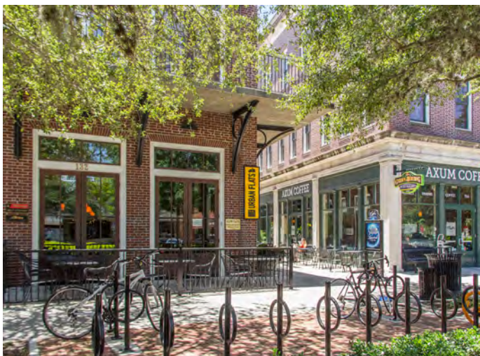
Downtown and neighborhood center can include larger mixed-use buildings.
