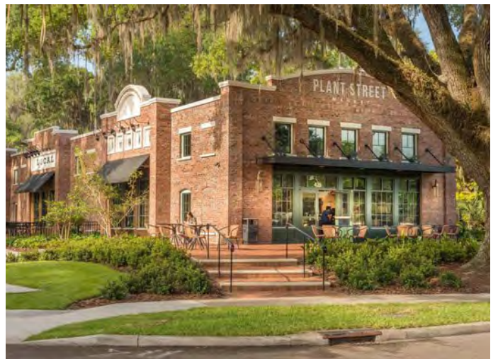
Neighborhood crossroads can include mixed-use buildings.
