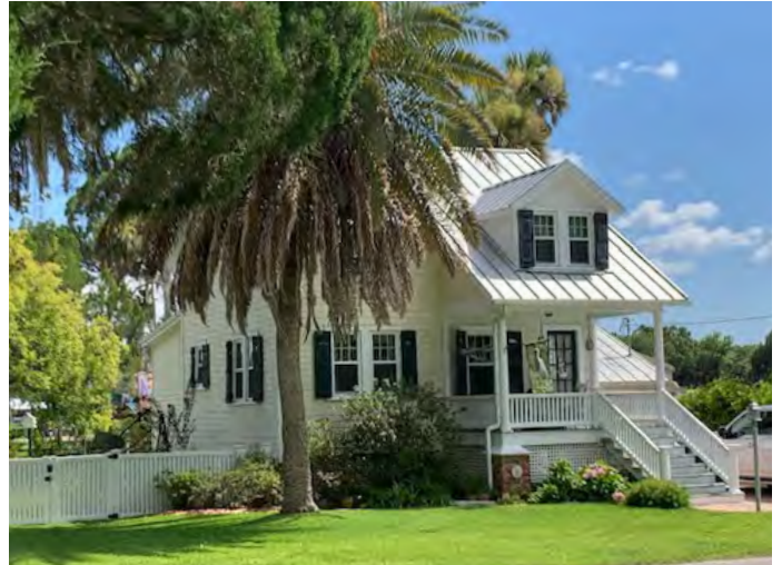
Existing traditional neighborhood character area in Crystal River.
