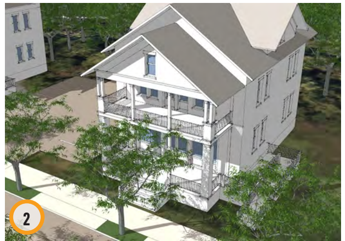
Porches provide a street-oriented frontage for buildings elevated to meet FEMA standards.
