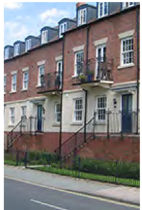
Examples of elevated buildings
