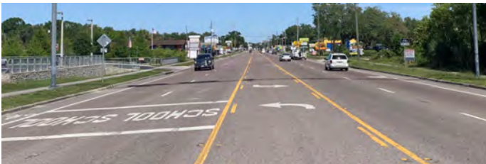
Photo of Highway 44 at NE 6th Ave looking east
