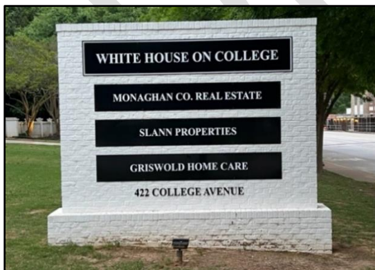
BASE WIDTH: 9'; BASE HEIGHT: 1' 6" SIGN WIDTH: 8'; SIGN HEIGHT: 6' TOTAL SIGN AREA: = 48 sf.
