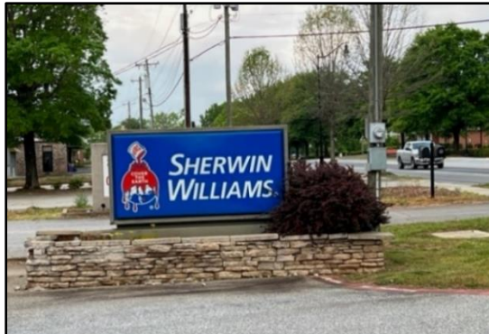
BASE WIDTH: 13'; BASE HEIGHT: 2' 6" SIGN WIDTH: 7'; SIGN HEIGHT: 4' TOTAL SIGN AREA: = 28 sf.
