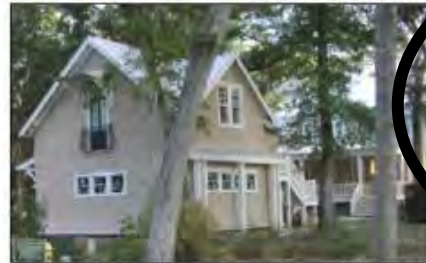
One-and-a-half-story carriage house with external stairway.
