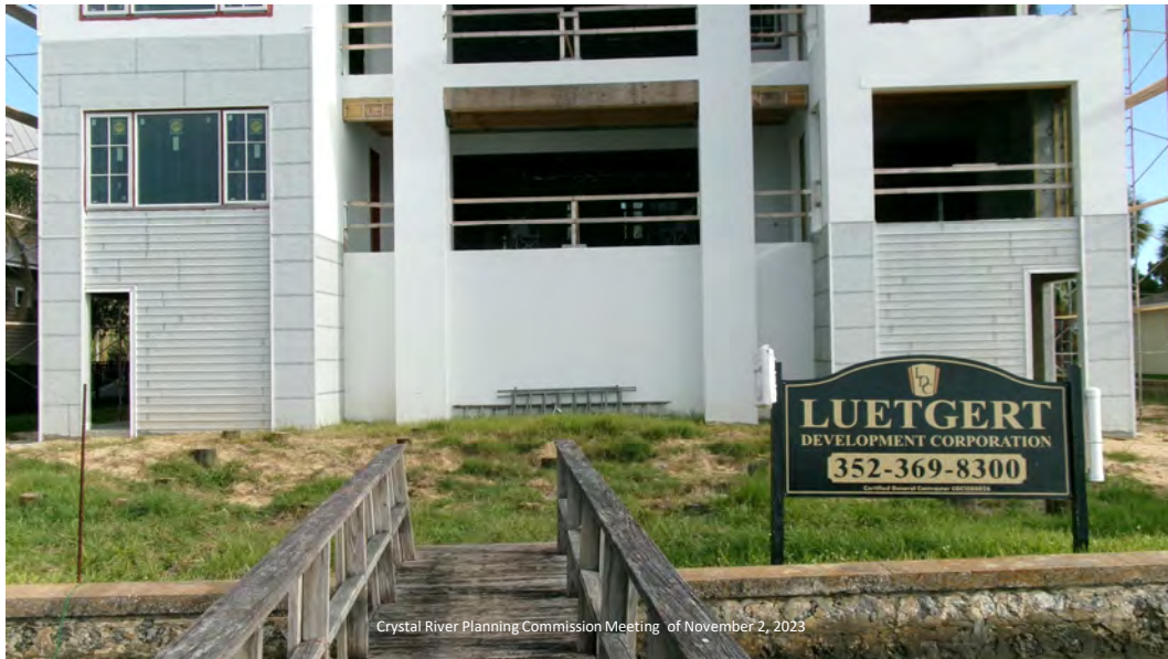
Looking from seawall to back of residence
