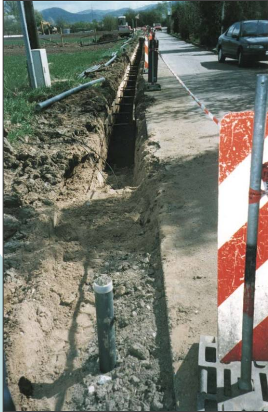
Force Main Pipe Installation
