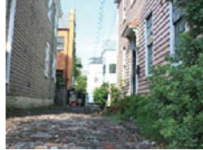
Primary frontage located upon a rear alley.
