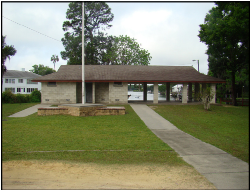
The restrooms block one of the best water-views in the park. Future improvements should remove this.
